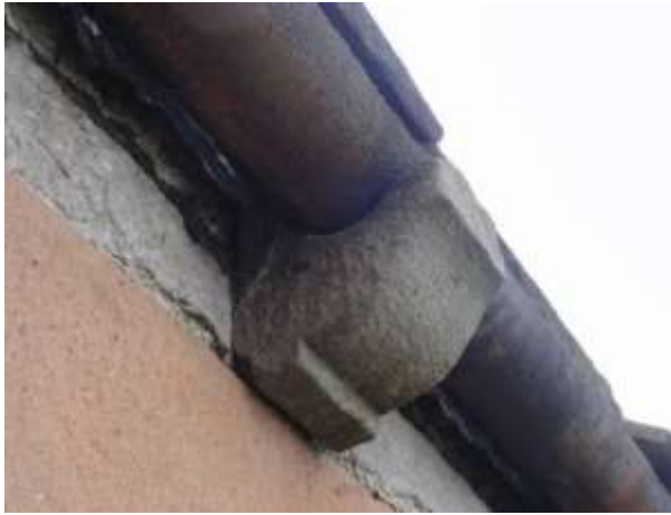
Stone support for a cast iron gutter on a historic barn (© Oldfield Design Ltd)
