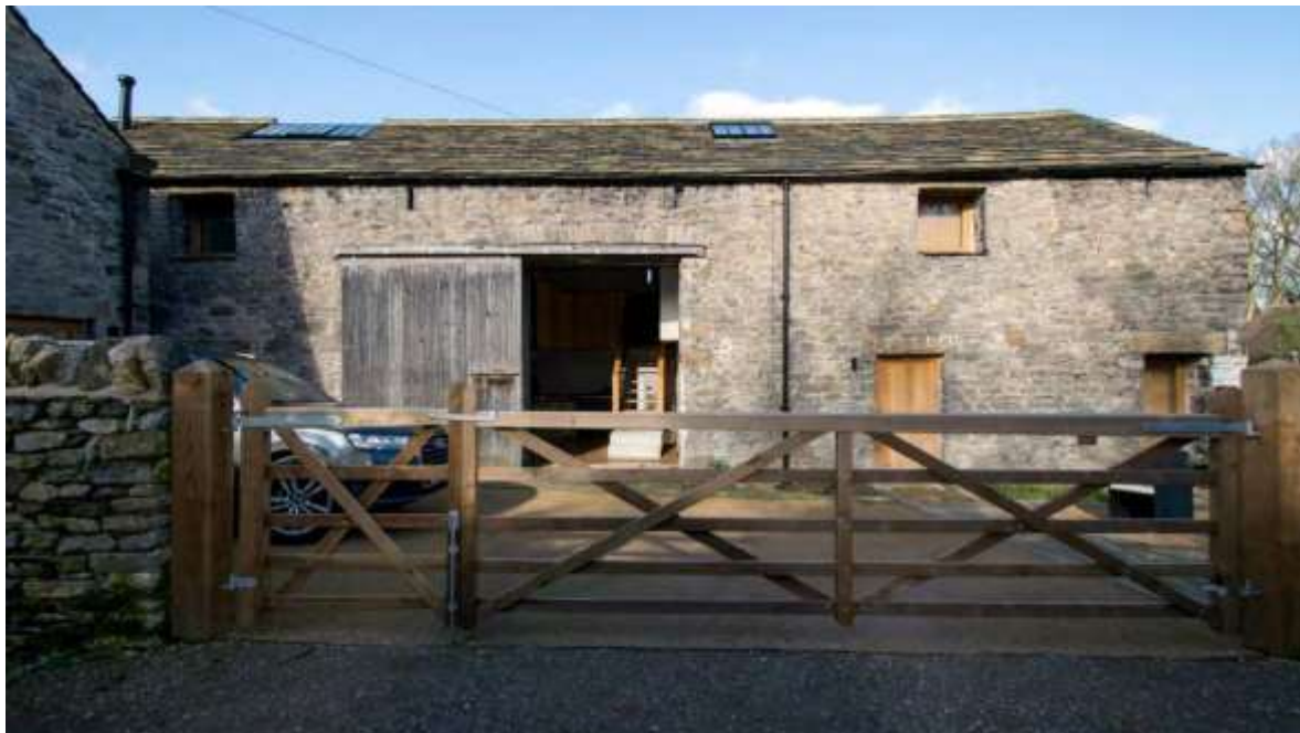
A barn after conversion to domestic use. The retention of the large sliding door and the careful use of existing openings with simple woodwork and internal shutters helps to maintain the agricultural character of the building. The interior is very modern but responds to the historic uses of space (© CE+CA Architects).
