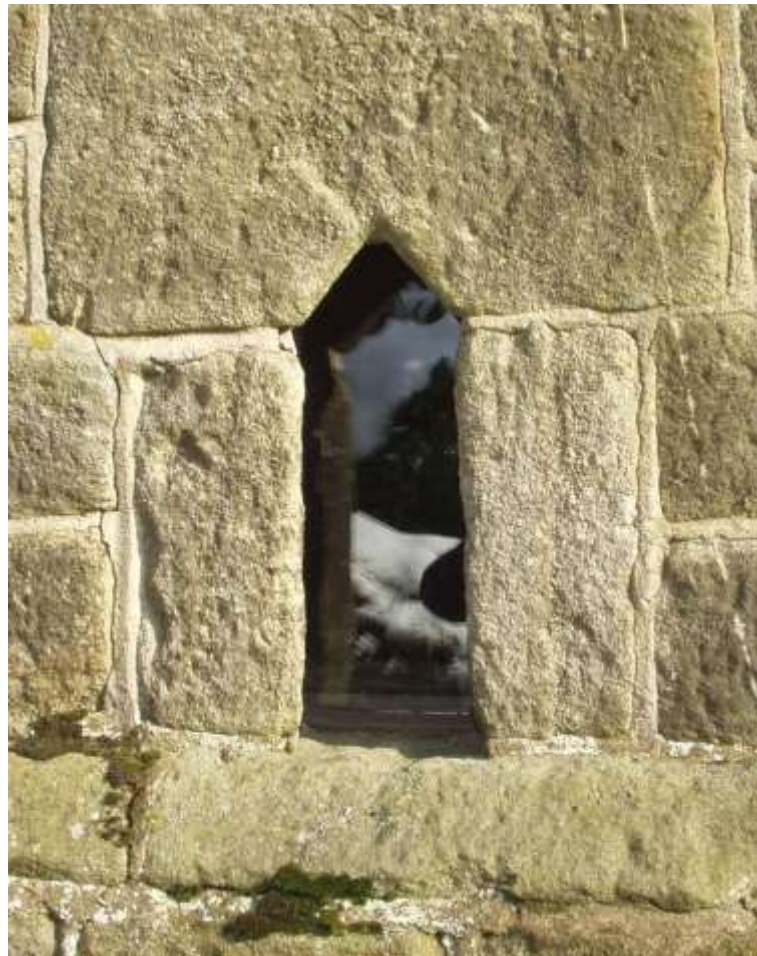
Glazing in a ventilation slot set well back into the reveal to reduce reflections, and fitted directly into the stone
