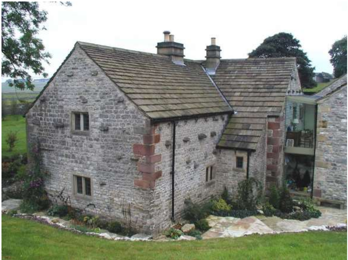
A glazed link filling in a narrow gap between a farmhouse and a former outbuilding at the rear allows each building to retain its own identity (© Bench Architects)
