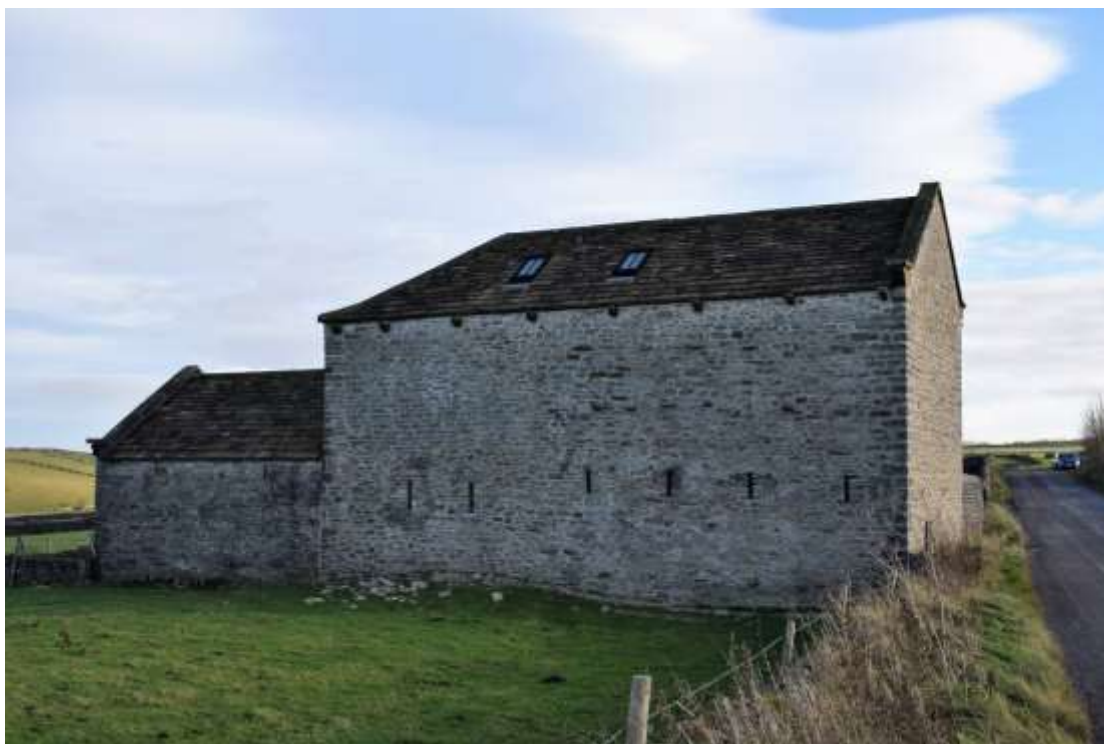
A barn after conversion – the solid-to-void ratio has been maintained. The only alterations on this elevation are two conservation rooflights and two additional vent slits to allow additional light to the interior. All the other original openings are on the opposite elevation (© PDNPA)
