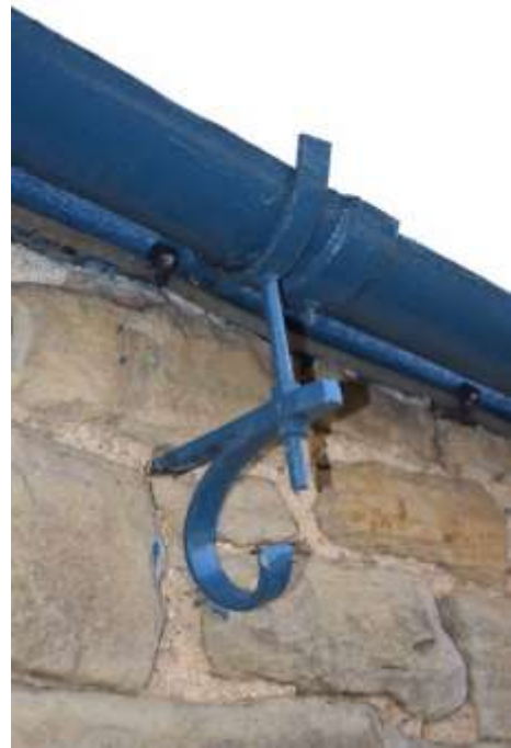
Metal bracket gutter support on a former smithy (© PDNPA)
