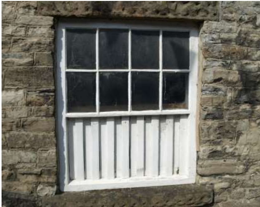
A traditional window with glazed upper and 'hit and miss' vents below (© PDNPA)
