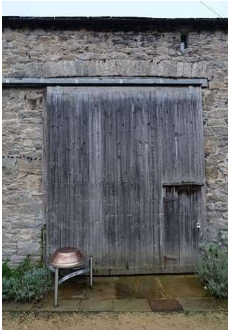
The 20 th -century sliding door on this threshing opening, although not part of the original building, has been retained and can be closed to cover the new glazed opening behind it. This maintains the agricultural feel of the converted barn and helps to tell part of the building's history. (© CE+CA Architects)
