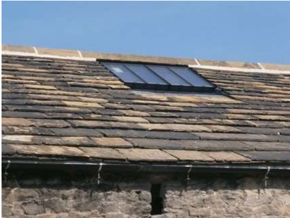
Industrial roof light set flush into a new stone roof along the ridgeline of this converted barn. The agricultural feel of the barn is maintained. (© PDNPA)
