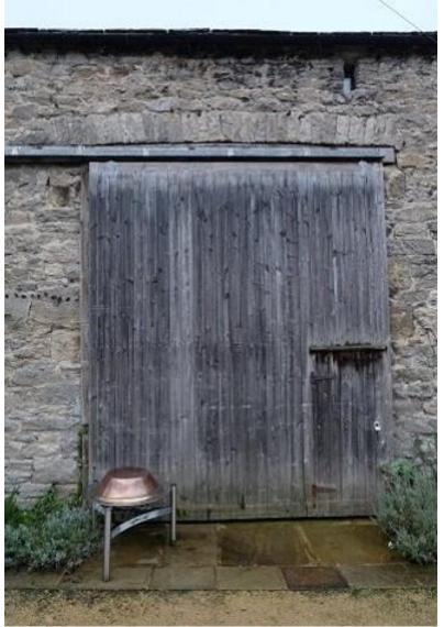
The 20<sup>th</sup>century sliding door on this threshing opening, although not part of the original building, has been retained and can be closed to cover the new glazed opening behind it. This maintains the agricultural feel of the converted barn and helps to tell part of the building's history. (© CE+CA Architects)
