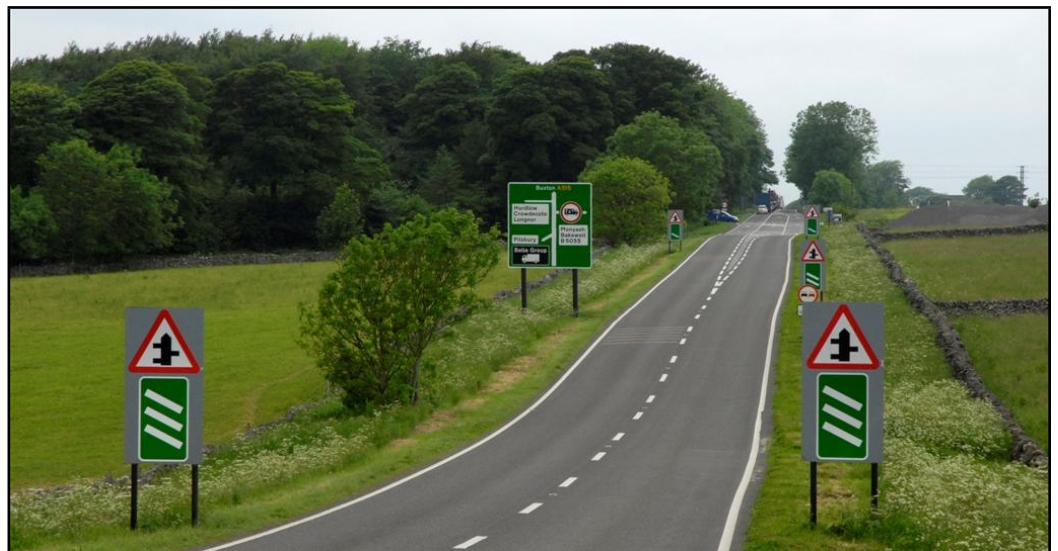
A515 at Monyash Junction - Further large junction count-down signs and large directional sign with black and passive-resistant support posts. Some of the signs also have grey backing boards, which makes them larger than without.
