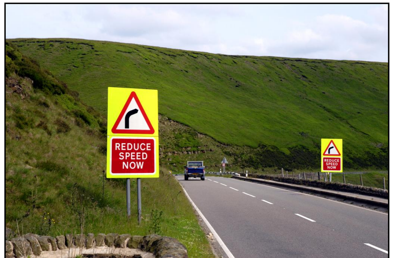
A57 Snake Pass - Further fluorescent-backed signs.
