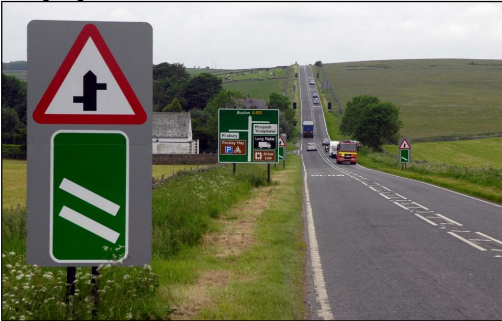
A515 at Parsley Hay - Large, obtrusive and potentially unnecessary junction count-down signs with black and passive-resistant support posts. Some of the signs also have grey backing boards, which makes them larger than without.
