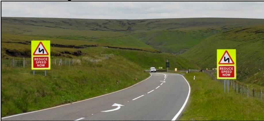
A57 Snake Pass - Highly obtrusive fluorescent yellow backed bend warning signs with VAS in the background.
