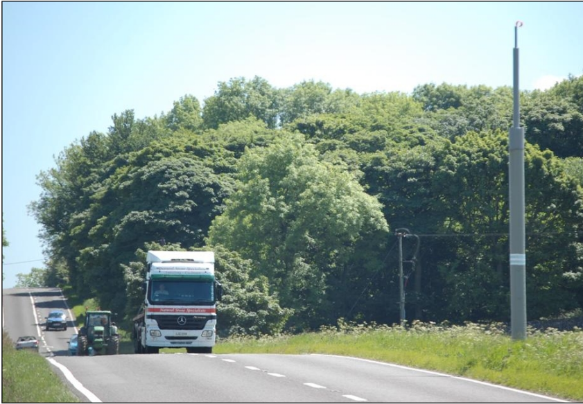
A515 – passive-resistant support post for VAS controversially installed late 2007, and unused since due to our objections.
