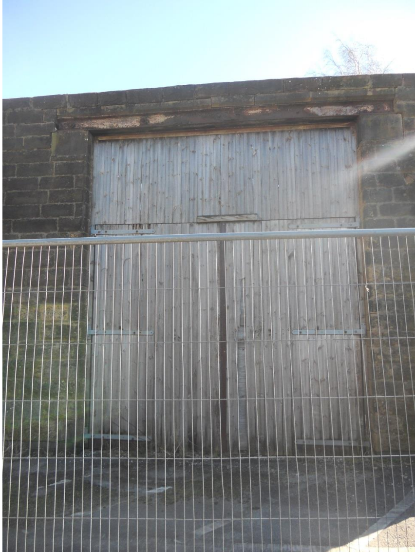
GOODS SHED DOORS WITH SAFETY FENCE
