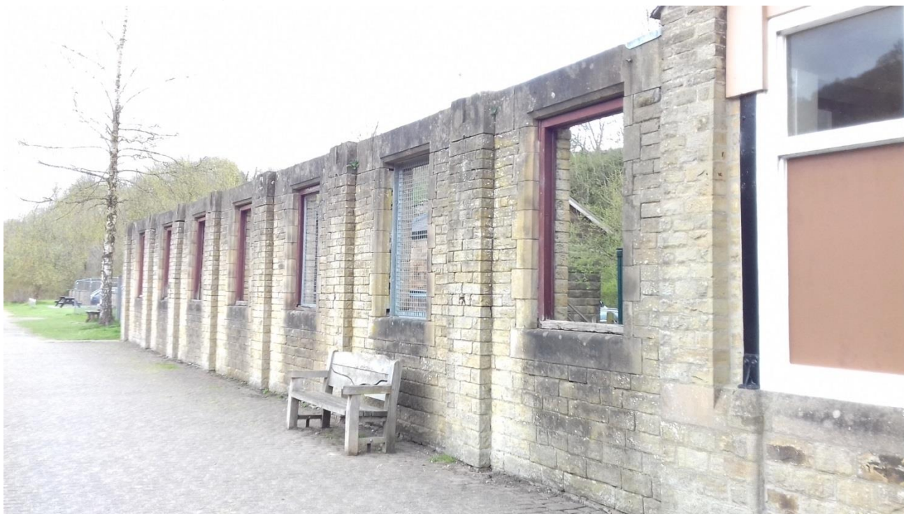
PLATFORM EXTERNAL FAÇADE WALL
