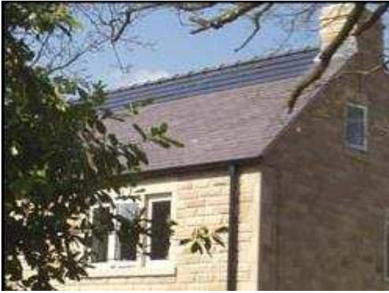
Photo 10. New build replacement dwelling, Curbar with simple arrangement of solar panels below the ridge
