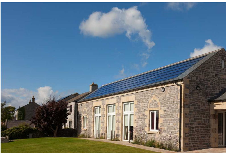
Photo 11. Over Haddon Village Hall
