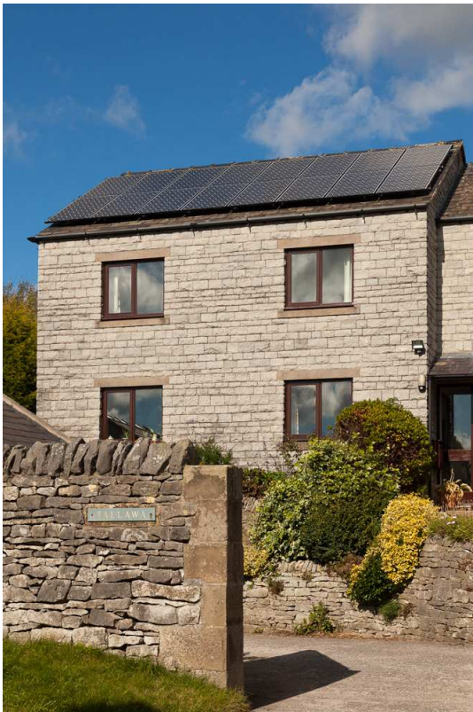
Photo 9. Retrofitted photovoltaics, Over Haddon
