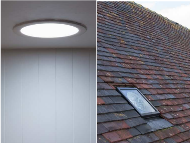
Figure 9 Sun Pipe – minimal impact on Grade II listed building
