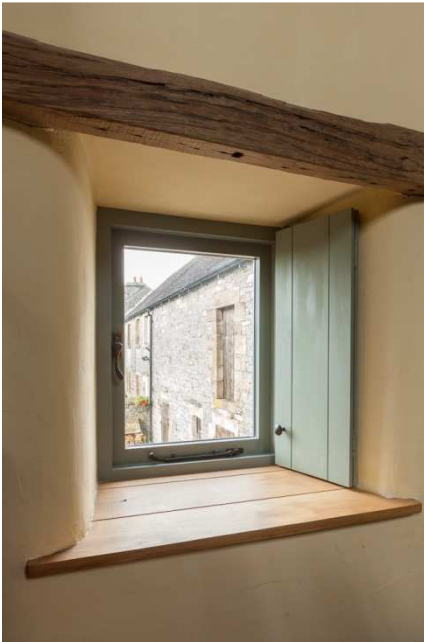
Figure 5 Insulated lime plaster walls conserve the internal appearance of the historic building whilst conserving energy. Home made internal shutters also conserve energy.
