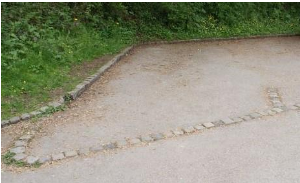
Figure 10.4 – Stone setts are used to delineate parking bays at Mapleton Lane car park near Ashbourne 49
