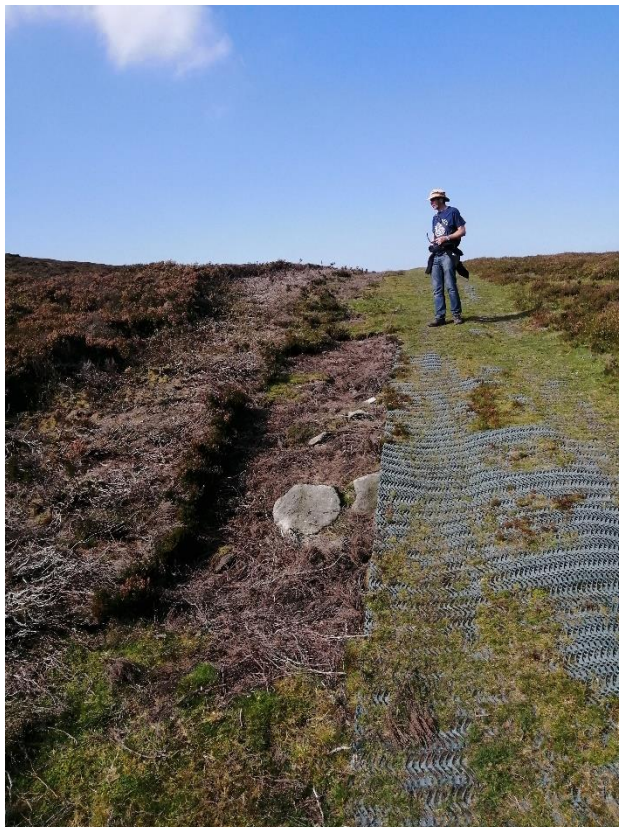
Figure 5 Heather brash cut alongside the track and used to repair eroding surfaces
