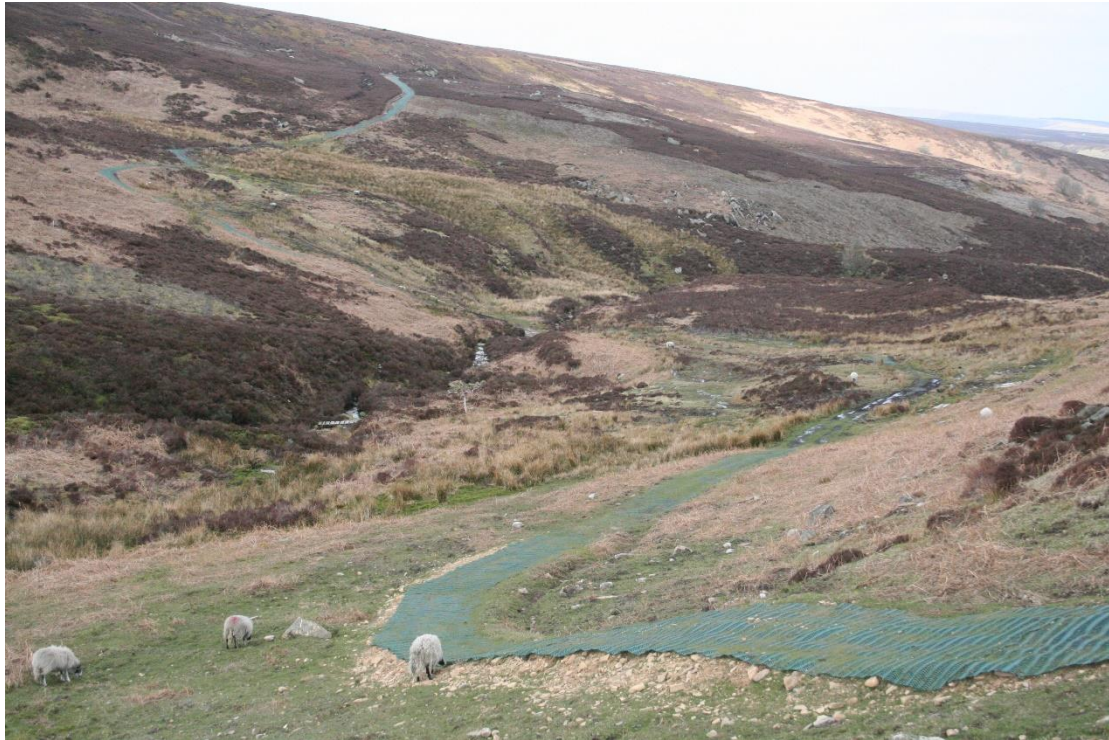
Figure 2 Midhope Moor track in 2018, showing that the track has been built up in this location.
