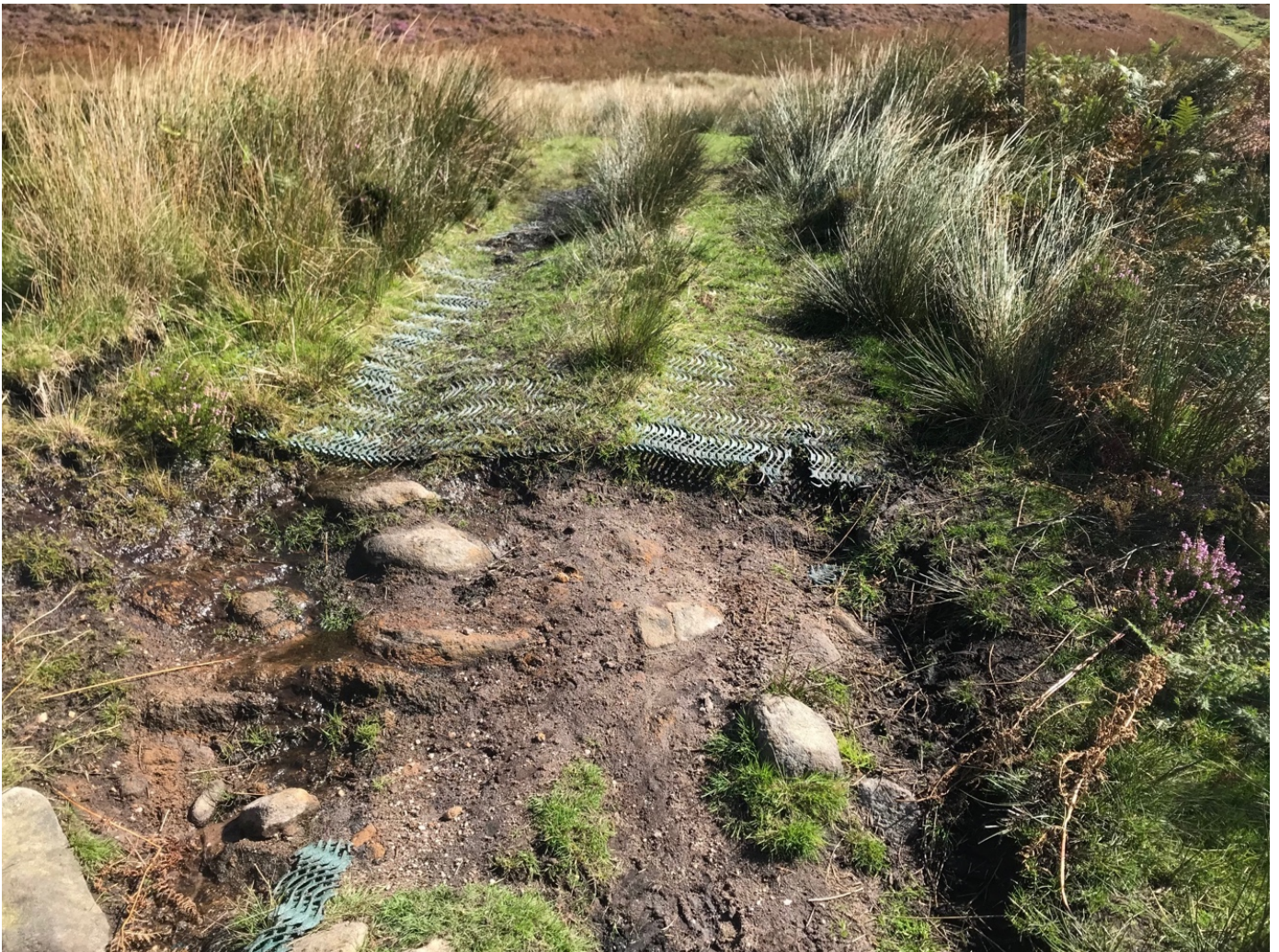
Photograph 1 Section of missing matting.
