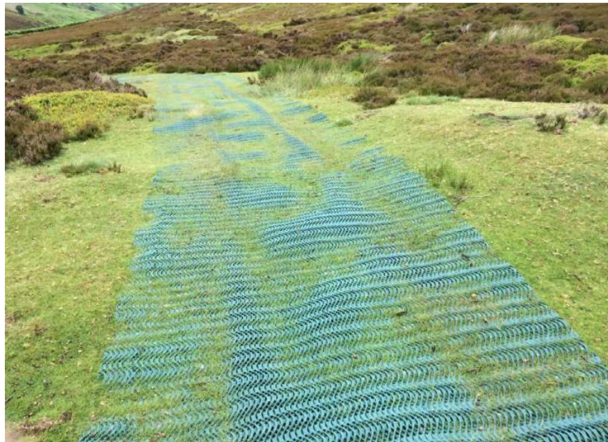
Photograph 8 After installation of appeal track July 2015 (Photograph by Davis & Bowring)
