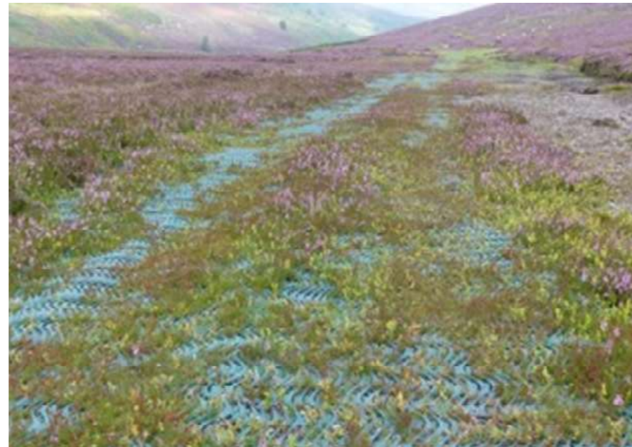
Photograph 9 After installation of appeal track September 2015 (Photograph by Davis & Bowring)
