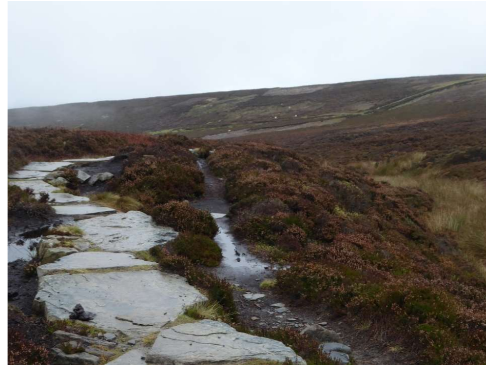
Photograph 16 View north along Cut Gate PRow Bridleway showing stone pavement section. (Oct 2020)
