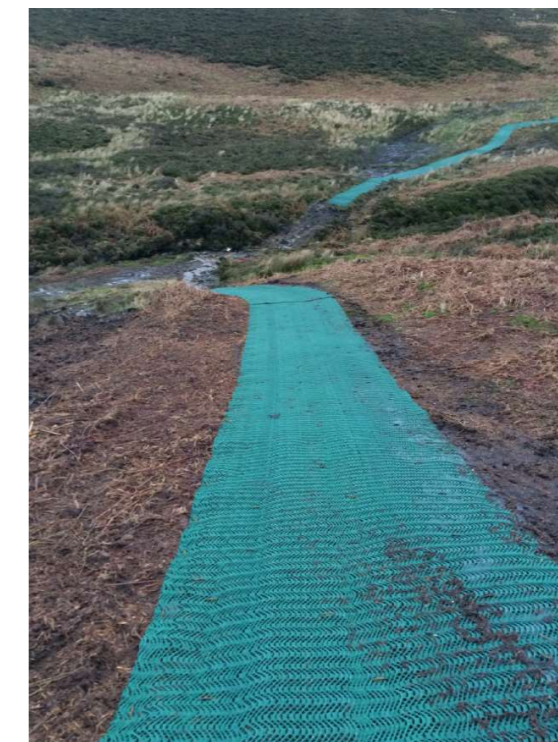
Photograph 10 After installation of appeal track July 2015 (Photograph by Davis & Bowring)
