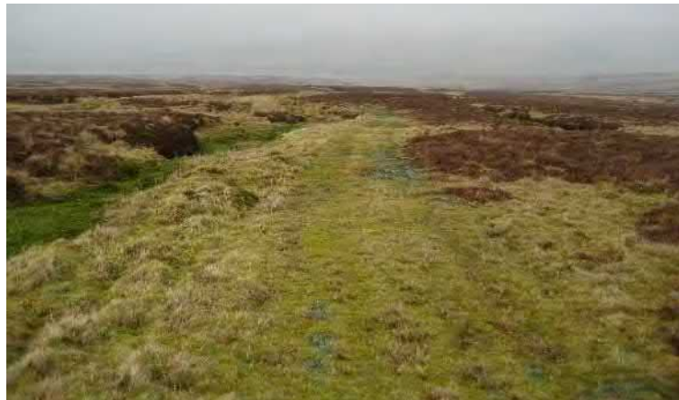
Figure 8.2 Plastic mesh track, approximately 1 year after installation on a working estate where vegetation was not cut prior to installation.
