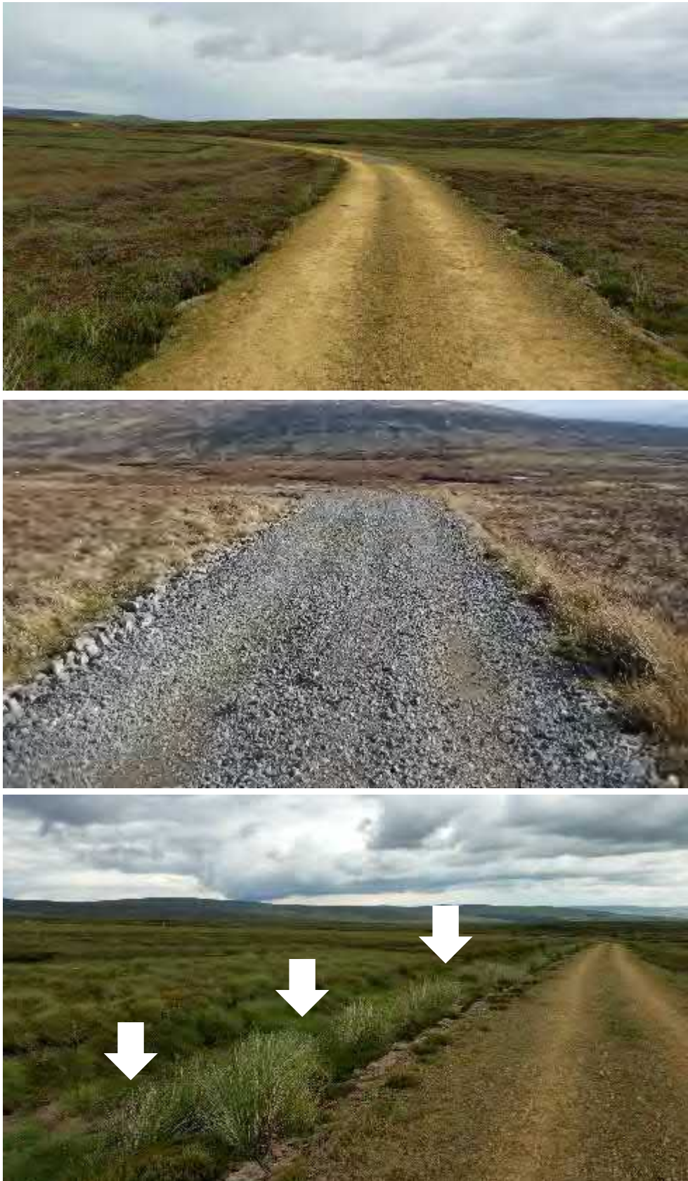
Figure 4.3 Types of stone track included in the upland survey. Top image of a floating sandstone track. Middle image of a limestone floating track. Bottom image example of a borrow pit track, with excavation adjacent to the track (left of photo) indicated by the white arrows.
