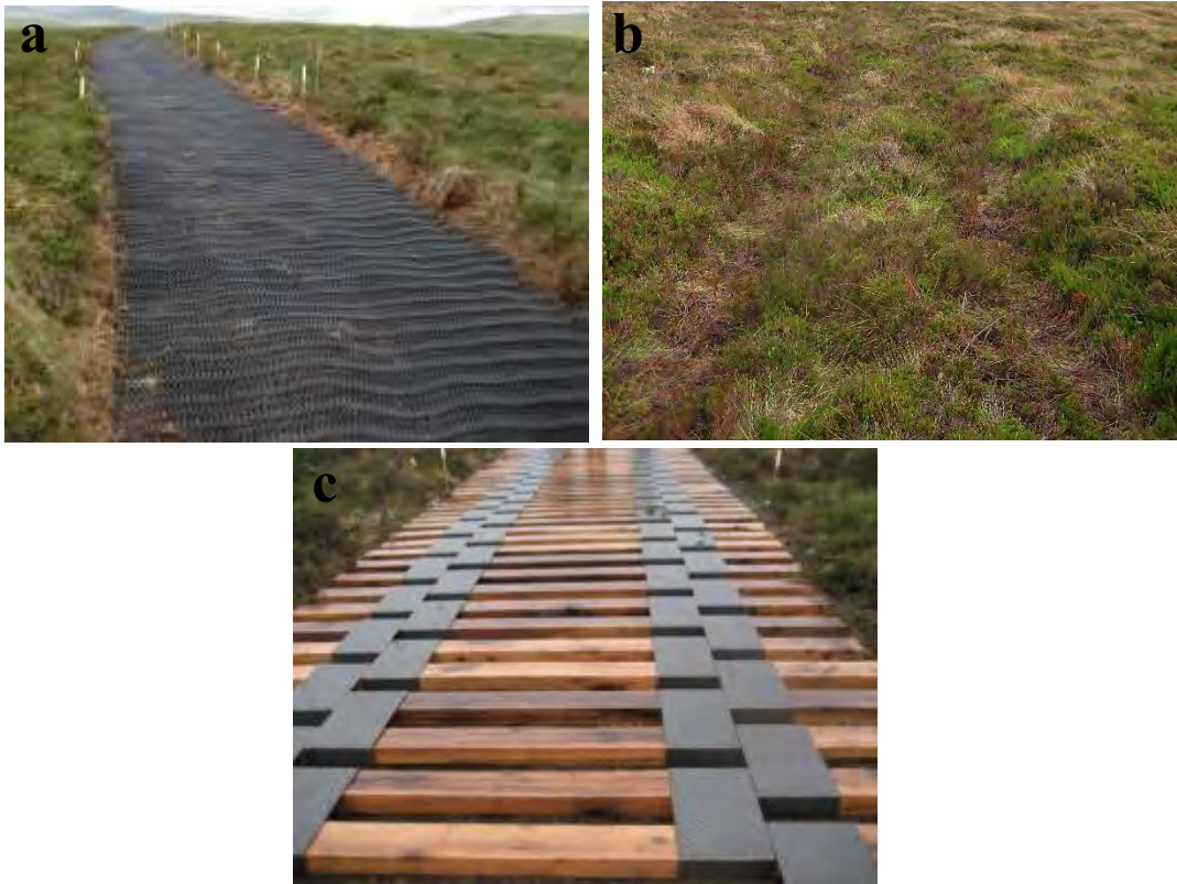
Figure 5.1 a-c Track types which have been included in this study. a) Plastic mesh, b) unsurfaced and c) articulated wooden.
