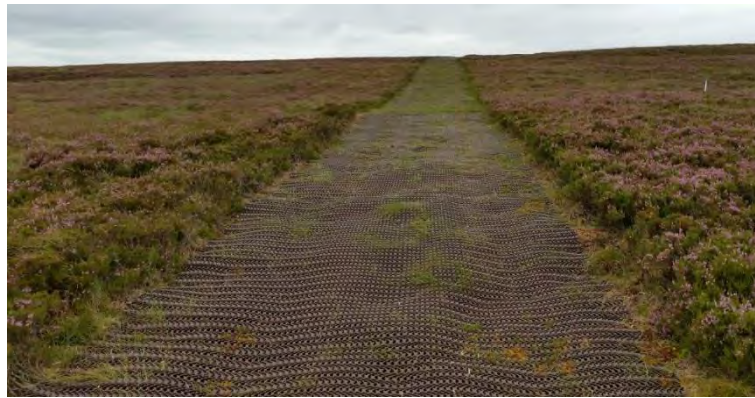
Figure 4.10 Plastic tracks installed perpendicular to the contours (i.e. straight up- and downslope) on working estates
