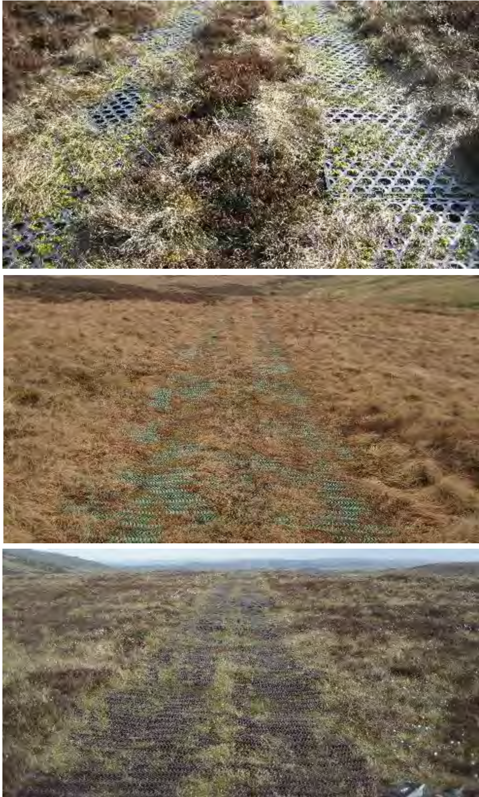
Figure 4.2 Types of plastic track included in the regional survey. Top image of plastic boards used in three study reaches. Middle image 2 m wide plastic mesh and bottom image 2.5 m wide plastic mesh, both constructed from UPVC.
