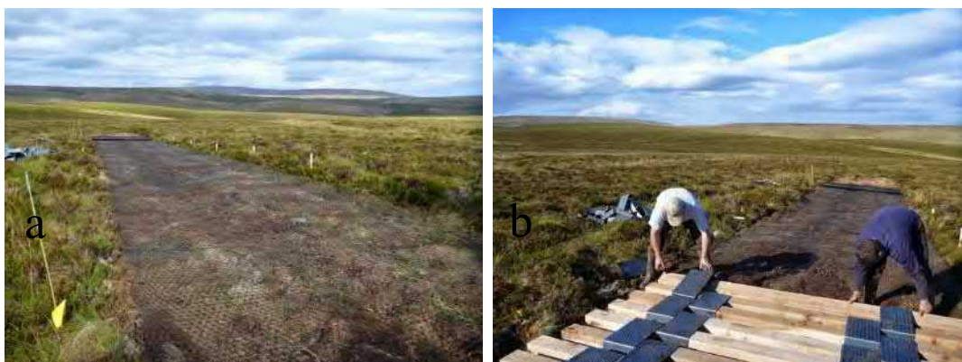
Figure 3.9 a-b Installation of wooden 4x4 track on Moor House NNR. a) Cut track route with thin plastic mesh and b) Oak beams laid along track route, connected with metal links. Photos courtesy of Andy Lloyd.
