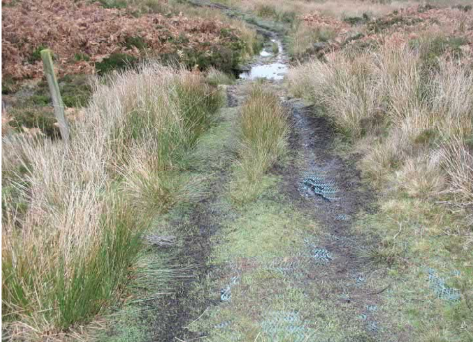
Photo 13 - looking west – incline down to the crossing point at Mickleden Beck The mesh is breaking up and sinking into the wet ground on slope.
