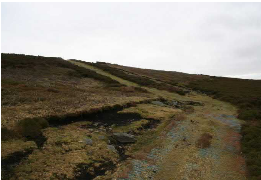
Photo 6 - looking south east along mesh track – towards the base of the incline Poor integration with surrounding land, with limited restoration of previous route. Limited vegetation establishment. The track is a prominent detracting feature which conflicts with landscape character.
