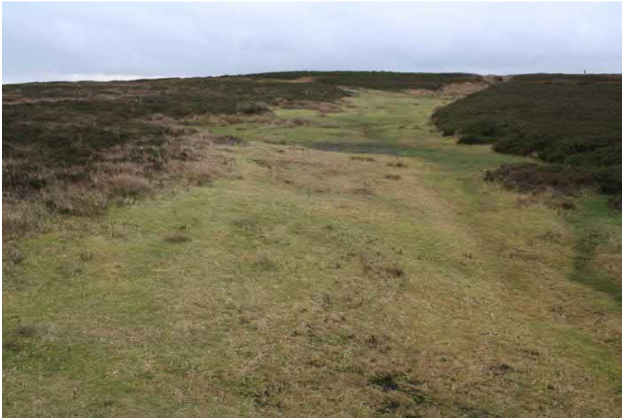
Photo 8 - looking south east along mesh track – at top of incline Better vegetation establishment (the mesh is not generally visible) with grass. This section is not visually inappropriate due to integration with surrounding grassed areas.
