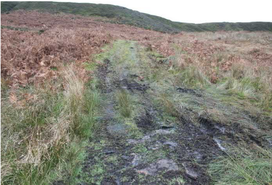
Photo 14 - looking west – climbing up from the crossing point at Mickleden Beck The mesh is again breaking up and sinking into the wet ground on the slope.
