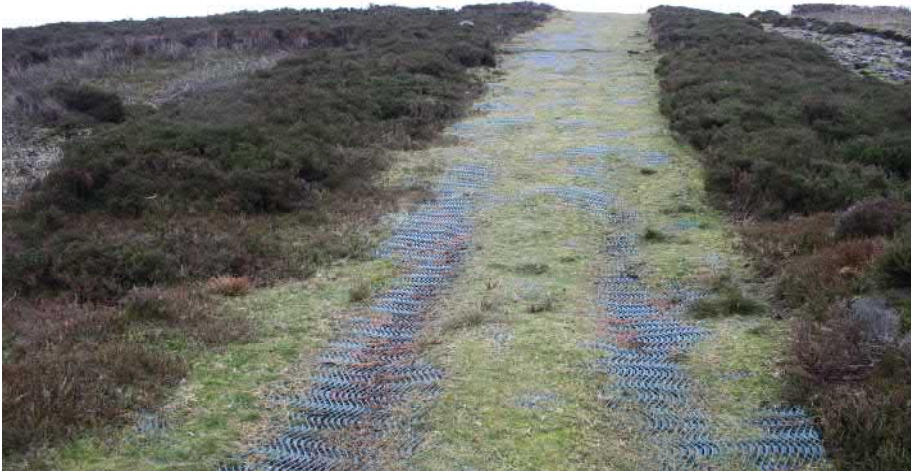
Photo 8 - looking south east along mesh track – at top of incline Better vegetation establishment (the mesh is not generally visible) with grass. This section is not visually inappropriate due to integration with surrounding grassed areas.
