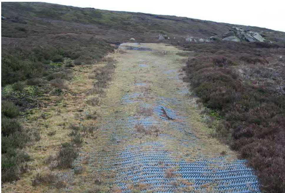
Photo 20 - looking north-west along mesh track – on incline Very limited vegetation establishment. Mesh clearly damaged and breaking up. Mesh poorly integrated with landscape and prominent through surrounding heather.
