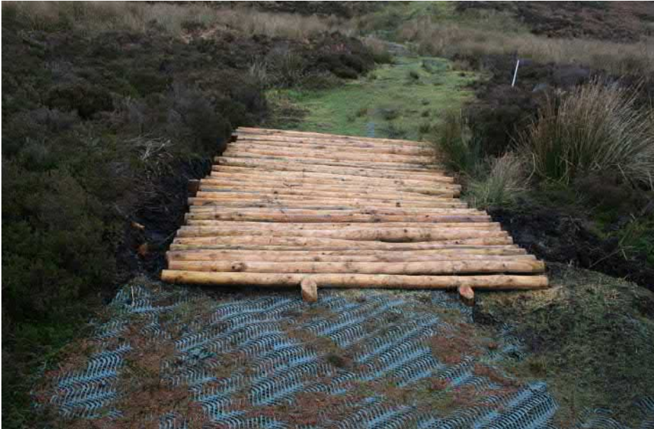
Photo 18 - looking north-west along mesh track Limited vegetation establishment and mesh again not coping with wet ground conditions. The log rafts are slightly less intrusive than the mesh (due to colour and better rush re-growth).
