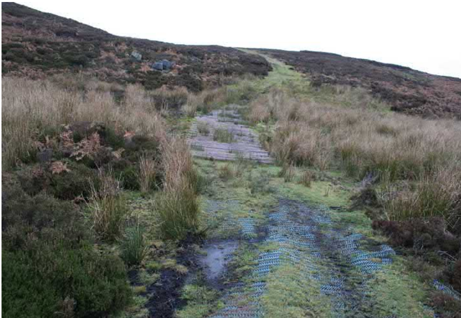
Photo 18 - looking north-west along mesh track Limited vegetation establishment and mesh again not coping with wet ground conditions. The log rafts are slightly less intrusive than the mesh (due to colour and better rush re-growth).
