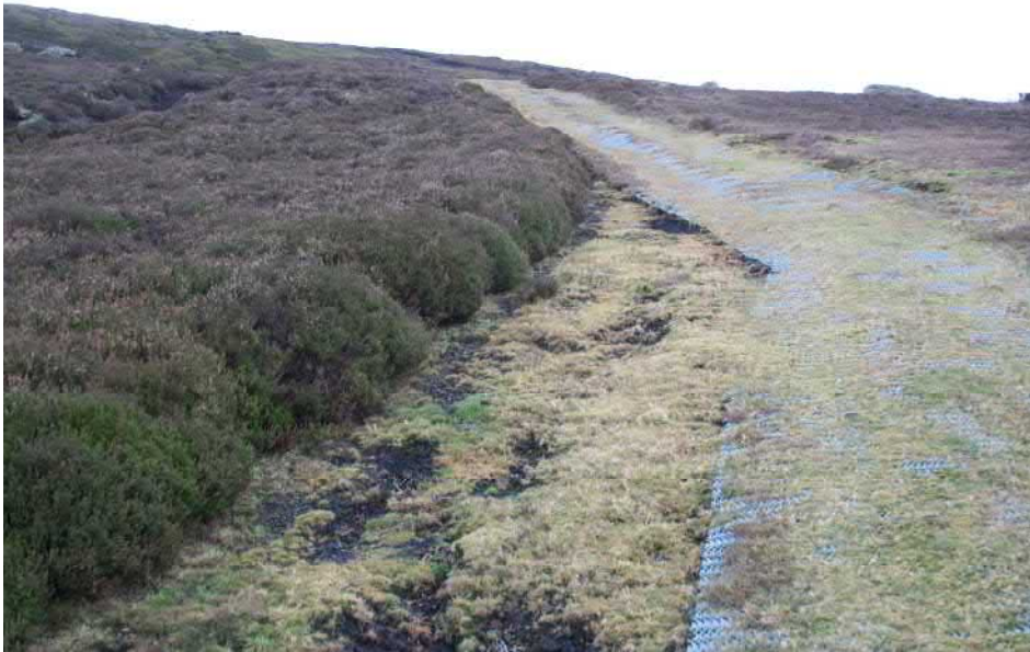
Photo 20 - looking north-west along mesh track – on incline Very limited vegetation establishment. Mesh clearly damaged and breaking up. Mesh poorly integrated with landscape and prominent through surrounding heather.
