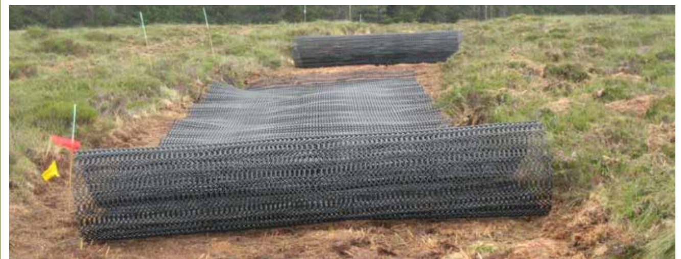
Fig 5. Mesh was rolled out.
