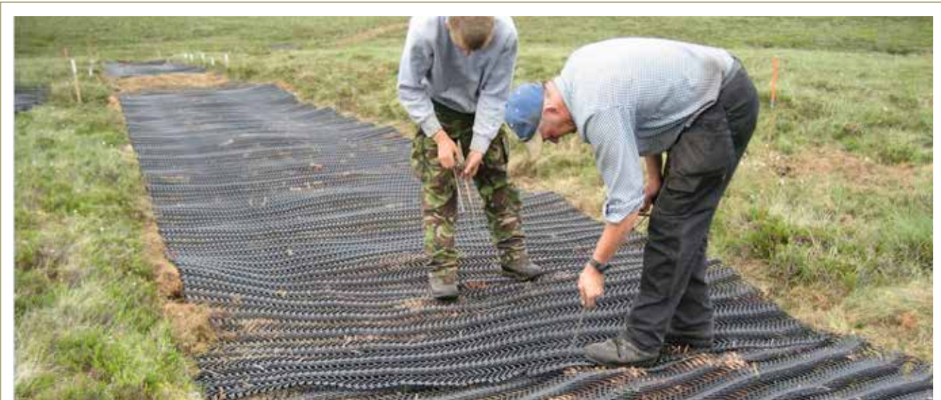
Fig 6. Mesh was pinned in place with 300mm steel U shaped pins.
