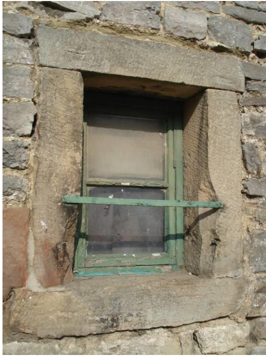
A like-for-like replacement of an historic window, including stonework repairs and new ironwork, based on evidence from the existing openings. (© Bench Architects)
