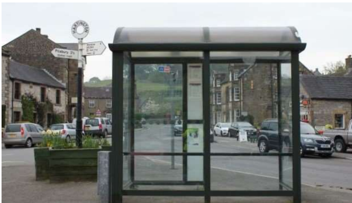
Figure 13.3 – Hartington Bus Shelter
