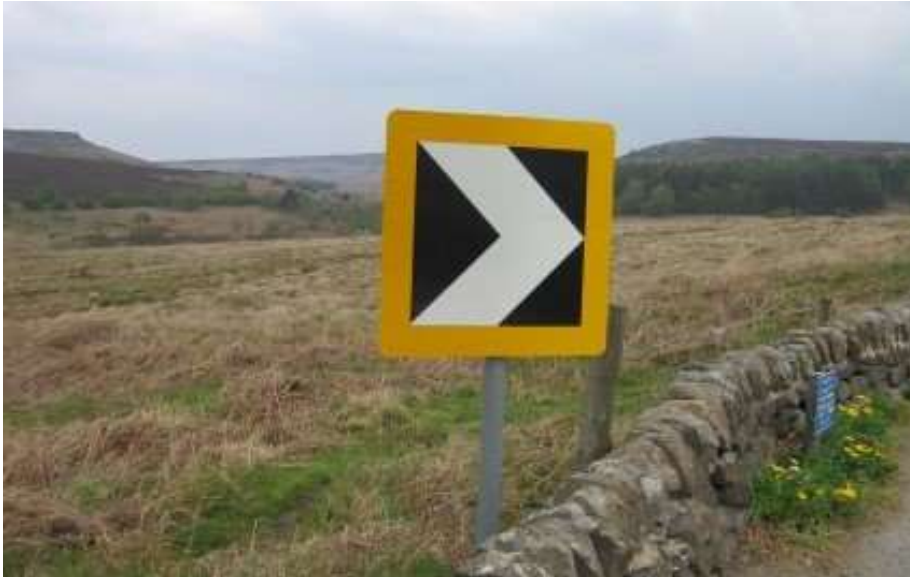
Figure 11.2 – Low Mounted chevron at Upper Padley, near to Longshaw
