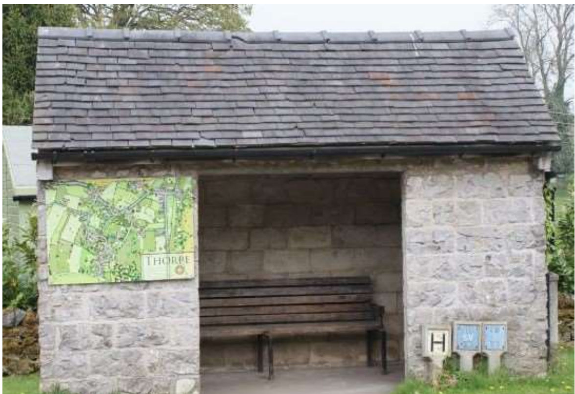
Figure 4.4 – Stone bus shelter in the centre of Thorpe
