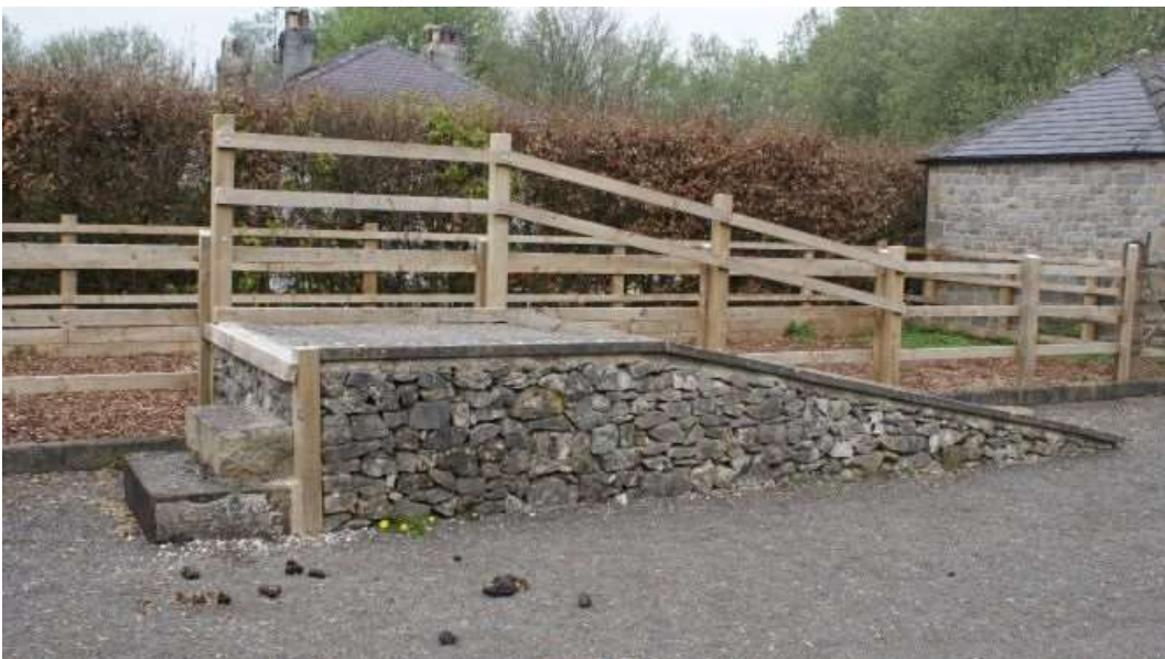
Figure 10.7 - Mounting ramp at Hartington Station Car Park
