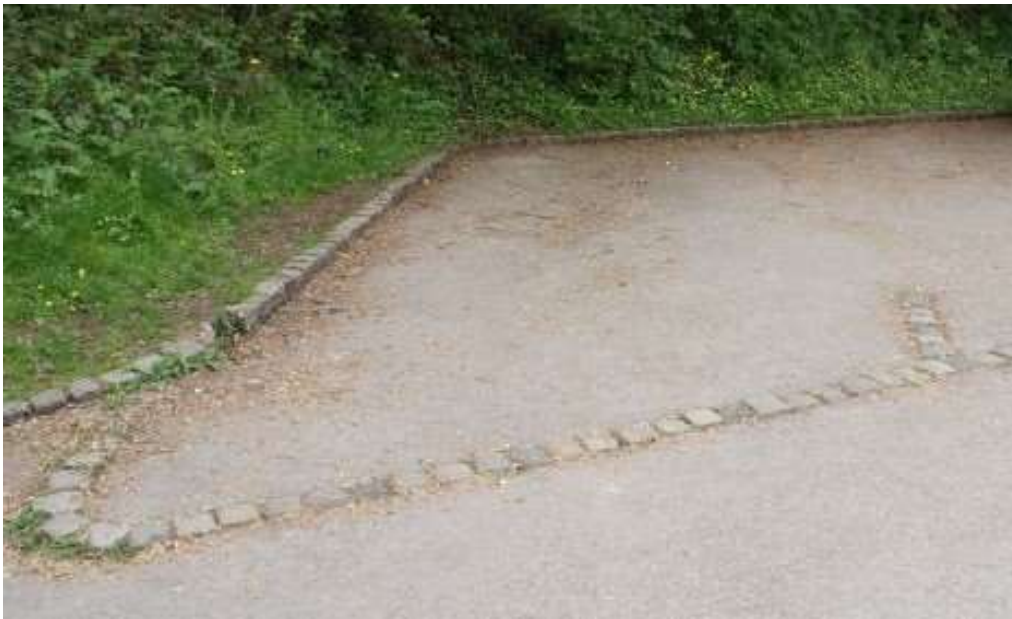
Figure 10.4 - Stone setts are used to delineate parking bays at Mapleton Lane car park near Ashbourne
