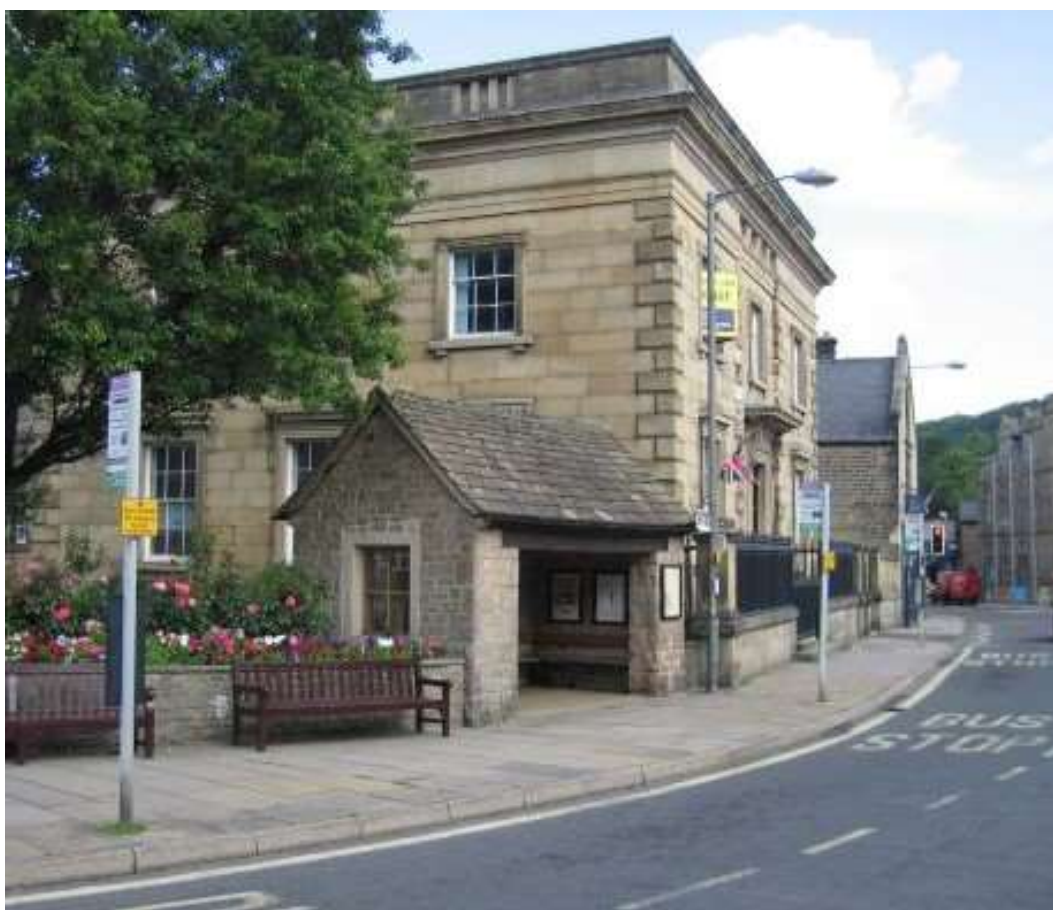
Figure 13.5 – Bus stop facilities at Rutland Square in Bakewell
