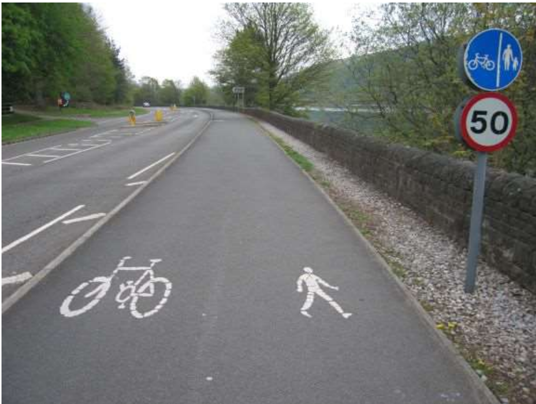
Figure 11.4 – Signed multi user routes adjacent to the highway at Hathersage (A6187, upper) and the Upper Derwent Valley (A57, lower)
