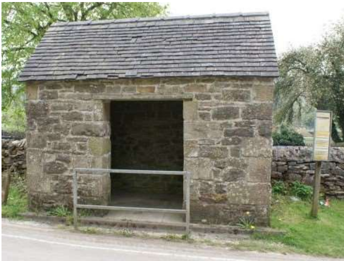
Figure 13.1 – Tissington Bus Shelter
