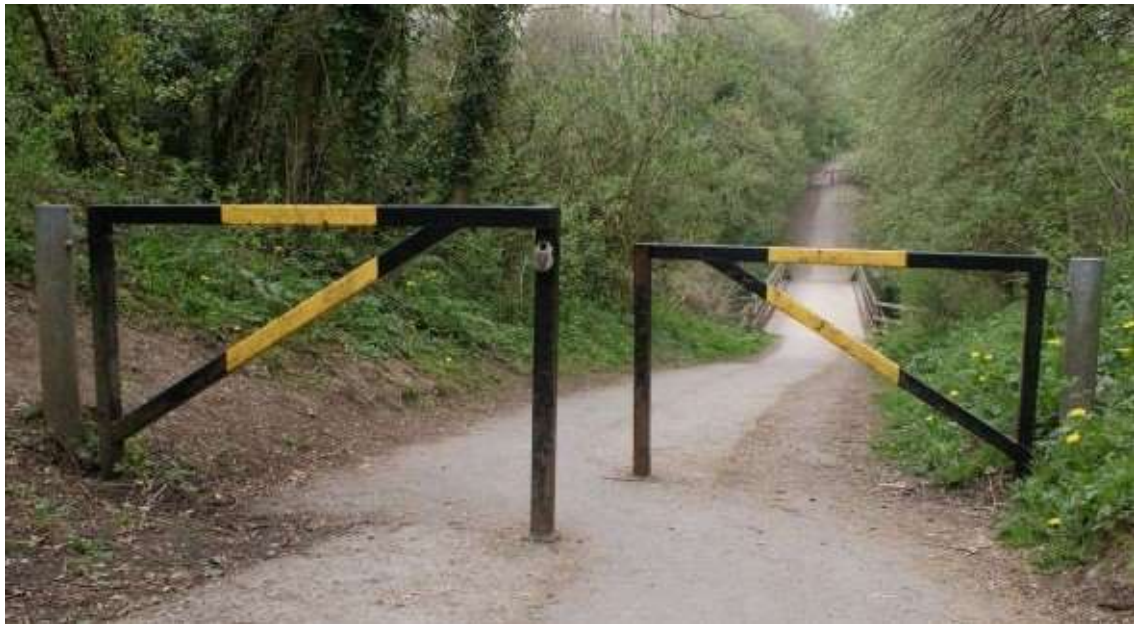
Figure 9.10 – Staggered gates to encourage slower cycling speeds on a ramp of the Tissington Trail
