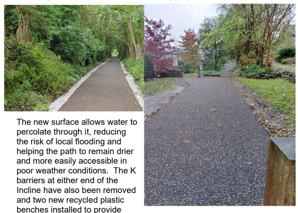
additional resting places along the route. This is the first time that we have used this type of material on such a substantial length of path (600m). The feedback received so far has been really positive and we will continue to monitor how weather resistant and hardwearing the new surfacing proves to be.
