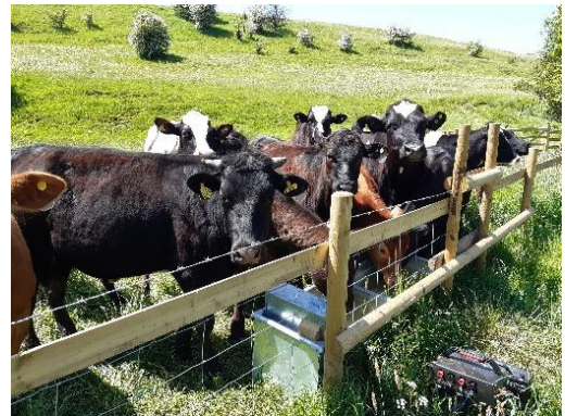
Photograph of solar powered water pump
