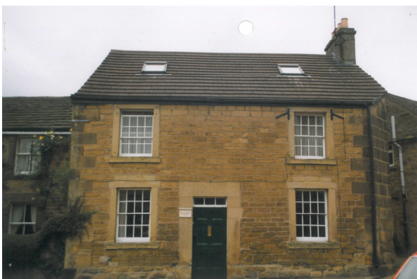
12 (left) BEFORE: a cottage in Eyam with concrete roof tiles and inappropriate modern rooflights.
