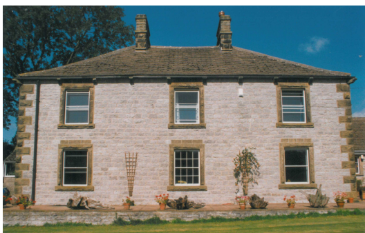
7 (left) BEFORE: modern, unsubdivided sashes in this early 19th century house near Foolow. (Tape has been added to one window to simulate the subdivision proposed.)
