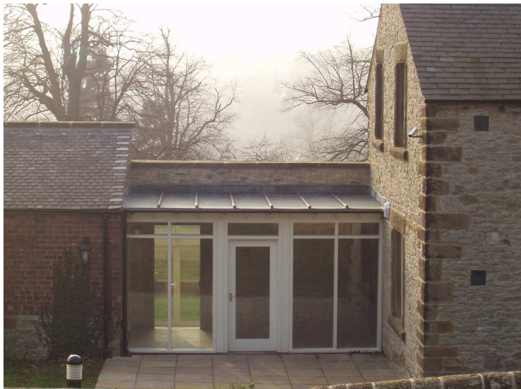
33 (left) A modern glazed link between two buildings. The minimum framing to the glass walls and roof allows maximum transparency and makes the link very unobtrusive. 34 (right) A more traditionally detailed, glazed link built against a high stone wall connecting two buildings.
