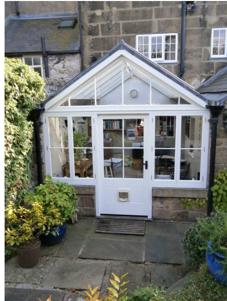
53 (right) A simple ridge-roofed conservatory on the rear of a listed building.
