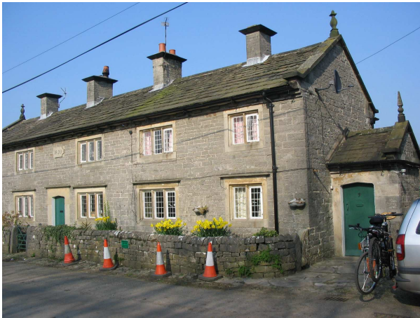
40 (left above) Enclosed, ridge roofed stone porch located on gable
