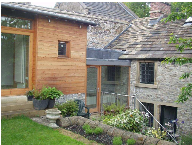
35 (left) A modern glazed link between the historic building and a modern timber clad extension. 35b (right) A traditional glazed link with simple vertical framing.
