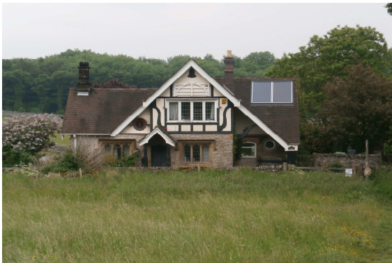
4 (left) Alterations over several decades have radically changed the look of what was a single storey toll house (originally one room either side of the central door).
