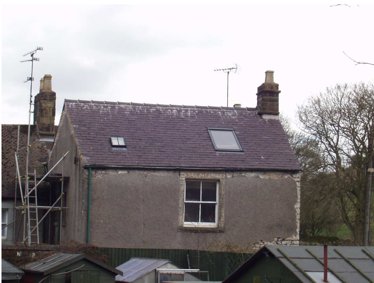
1 (left) Size matters. The small conservation rooflight on the left looks much more appropriate on this traditional building than the oversized, modern rooflight on the right.
