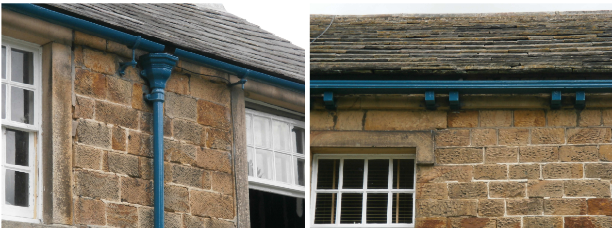
The two types of traditional rainwater goods: 17 (left) Cast iron guttering on rise and fall brackets. 18 (right) Timber trough guttering on timber corbels.
