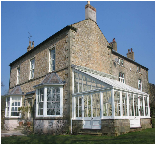
52 (left) A lean-to conservatory on the gable of a 19 th century house
