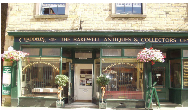
56 (above) Permanent bars fitted inside the window (King Street, Bakewell)
