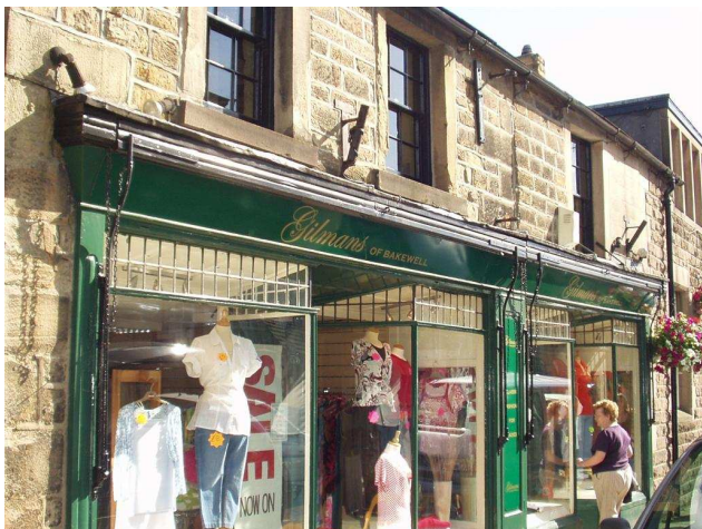
38 Projecting cornice incorporating traditional blind box
