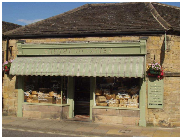
39 Original blind mechanism still in place
