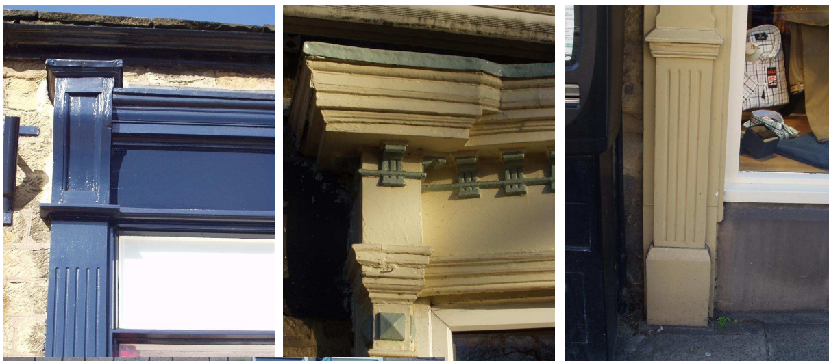
23-25 (above) Fascia, pilaster and plinth details often have Classical precedence
